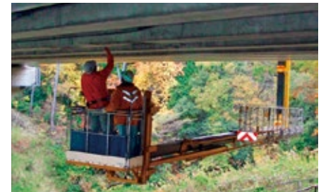
Inspection of a bridge
